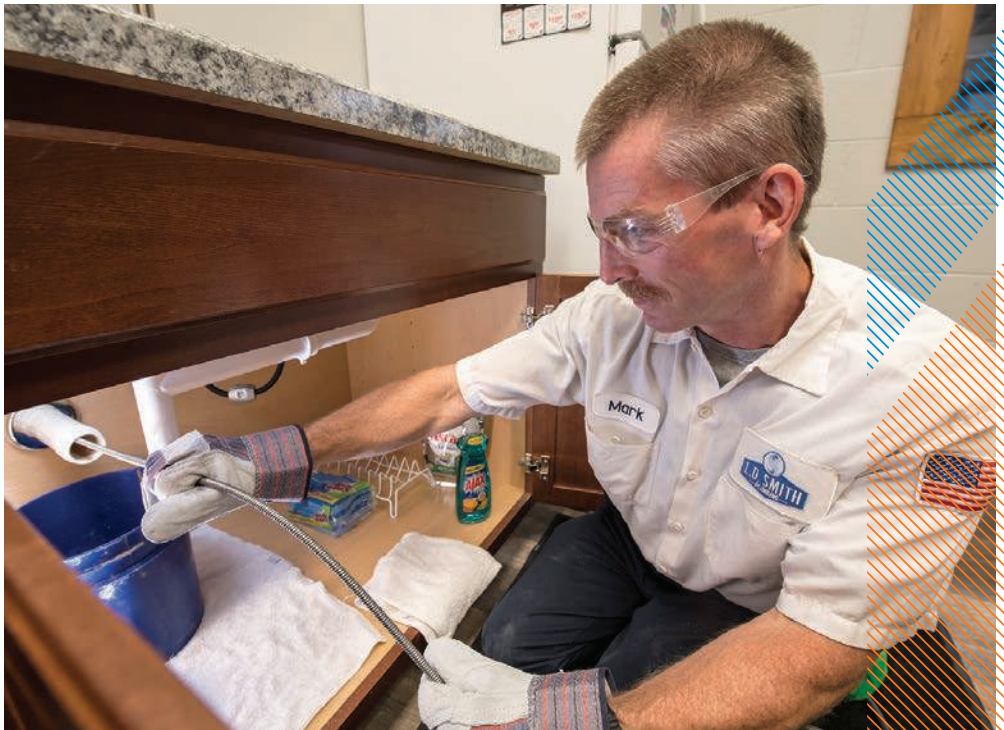
▶ Plumber Mark Lambert cleans out a sink drainpipe with a Spartan Tool 100 machine with a 5/16-inch 75-foot long cable. The Spartan 100 machines are equipped on every service truck.
