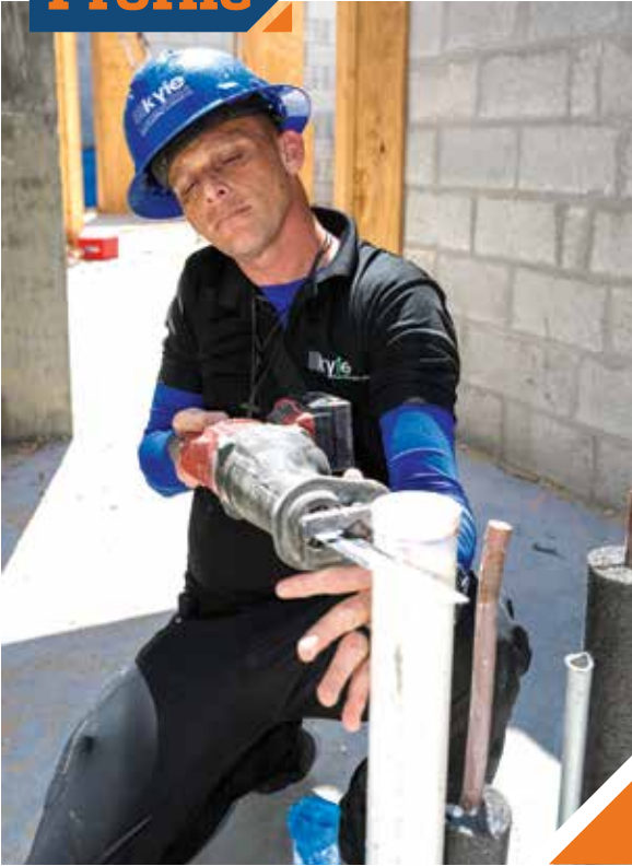
◀ General manager Louie Embroz carefully trims a pipe on a home project using a Milwaukee Tool Sawzall.
